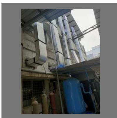
GI Ducting Installation Services
