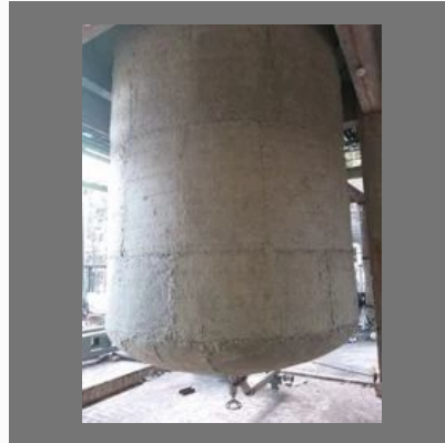
Hot Insulation Services
