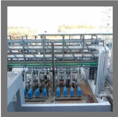
Armaflex Nitrile Rubber Insulation Work
